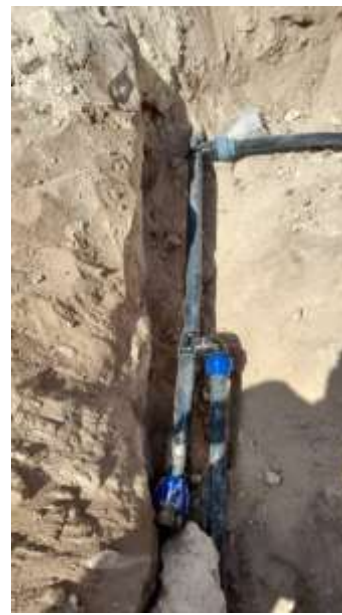
Raccordement aux maisons
